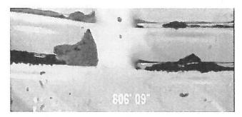
Well 6 has iron corrosion due to dissimilar metals casing materials, which may affect the remaining life of the well, although there is only a minor occurrence of rust particles in the water produced. The well casings in wells 2, 4, and 5 are constructed of stainless steel and do not exhibit corrosion. The wells have lost some of their original capacity and the well pumps are oversized for the sustainable yield.
